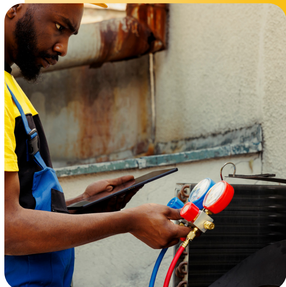
Technician reading pressure levels on manifold gauges. © Shutterstock
