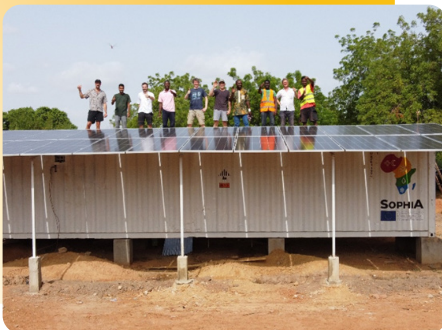
Inauguration of SophiA containers at Dr. Sedego Hospital in Léo, Burkina Faso.
