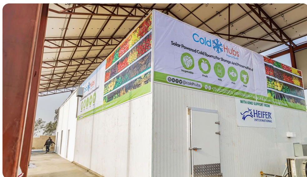
ColdHubs, Cooling as a Service in Nigeria: a walk-in, modular, solar-powered R290 cold room for storing fresh produce in Nigeria © ColdHubs
